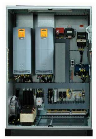
Illustration shows typical panel including AC690+ with AFE and additional system components.
